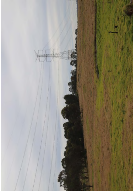
Photo 2. View west from within the south east part of the site.
